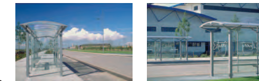
⑥ Bus Shelter
