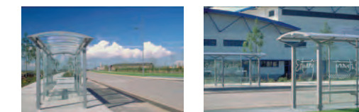
⑥ Bus Shelter
