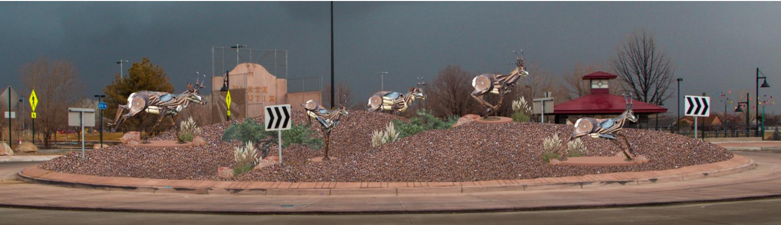
View Looking NE
