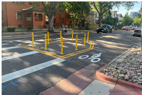
Retrofit Partial Closure
