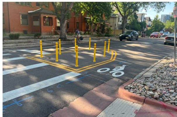
Retrofit Partial Closure
