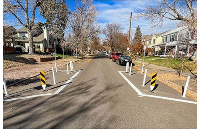
Retrofit Choker (source: City of Denver, Colorado)
