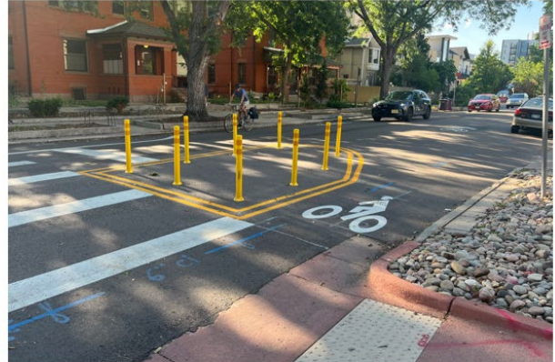
Retrofit Partial Closure
