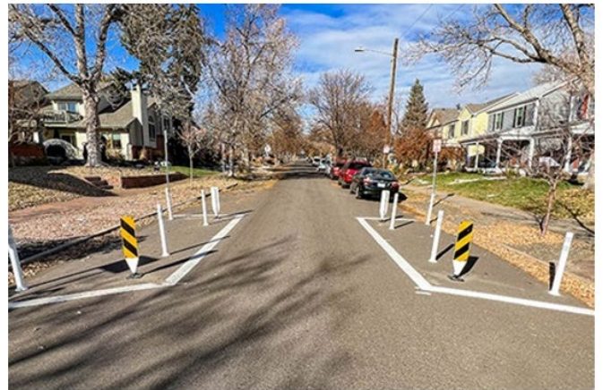
Retrofit Choker (source: City of Denver, Colorado)
