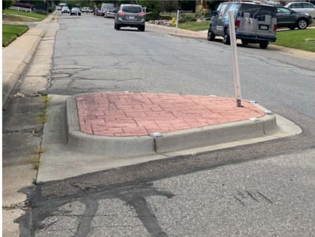
Permanent Chicane (source: City of Denver, Colorado)
