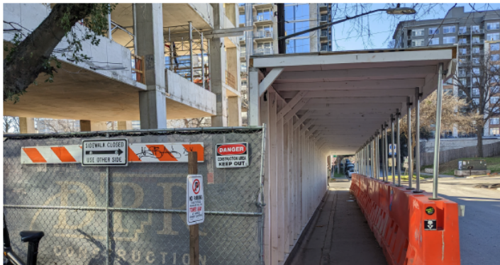
FIGURE 43: EXAMPLE OF COVERED WALKWAY AT CONSTRUCTION SITE
