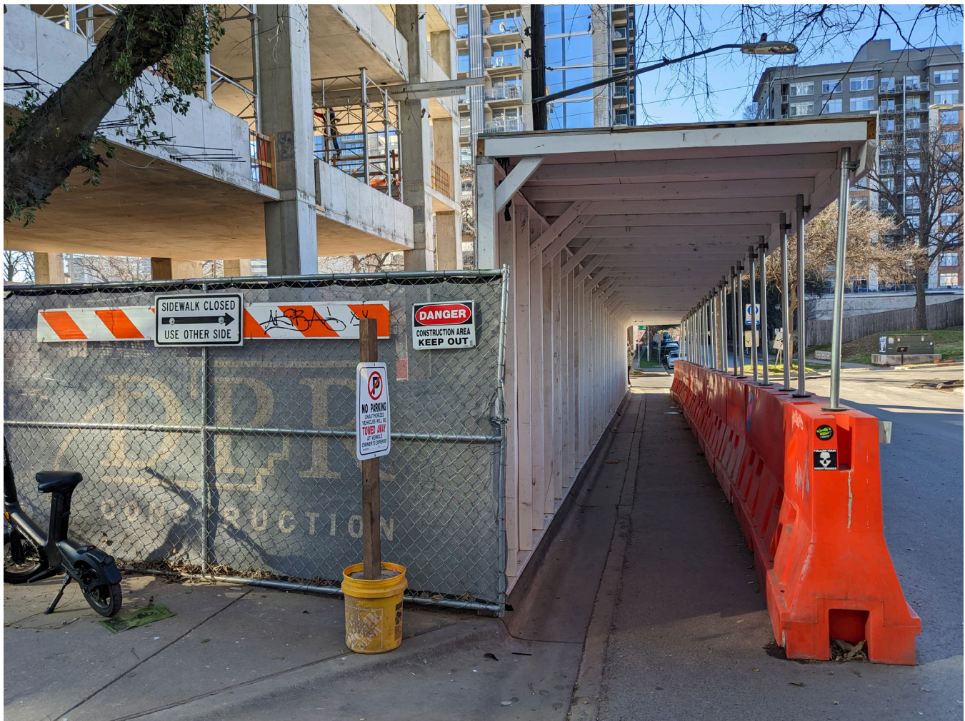
FIGURE 43: EXAMPLE OF COVERED WALKWAY AT CONSTRUCTION SITE
