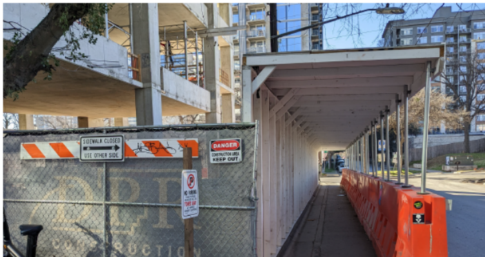
FIGURE 43: EXAMPLE OF COVERED WALKWAY AT CONSTRUCTION SITE
