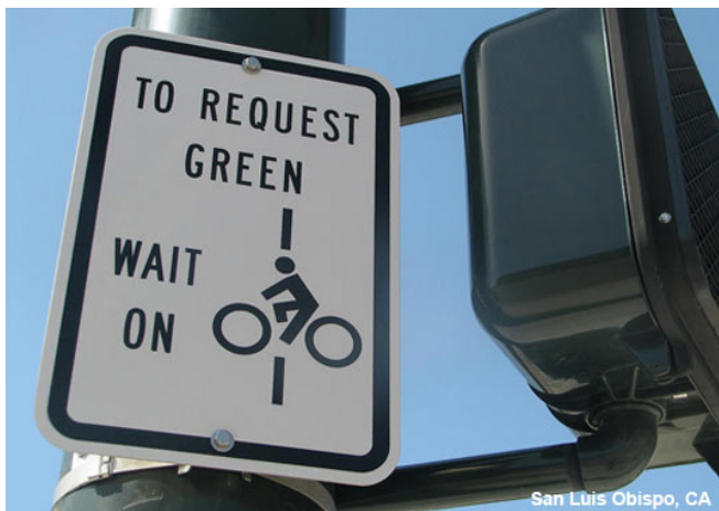
FIGURE 27: BIKE DETECTION AT SIGNAL
