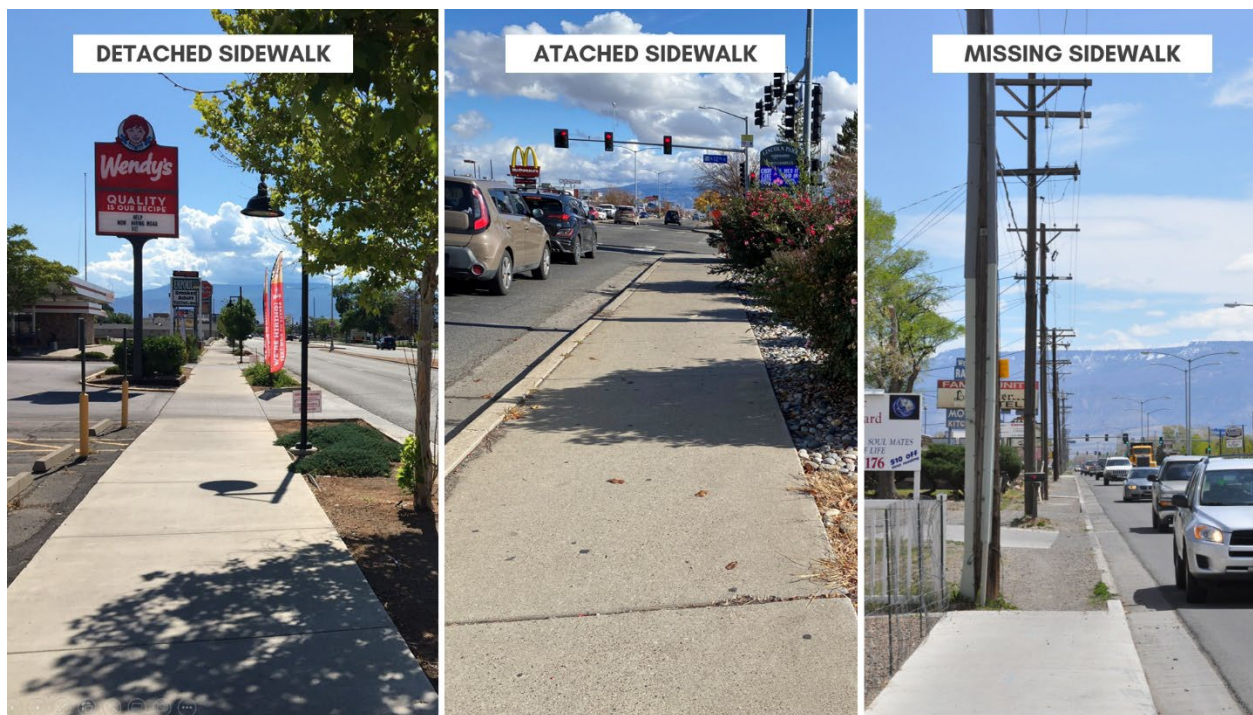
FIGURE 2: SIDEWALK CONDITION EXAMPLES
