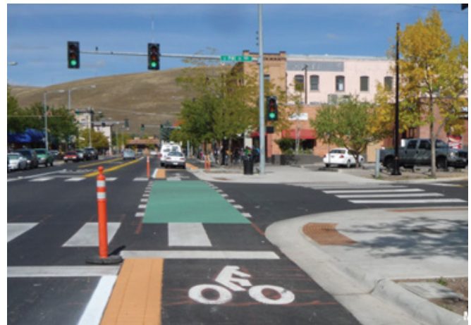
FIGURE 28: RECESSED STOP BAR
