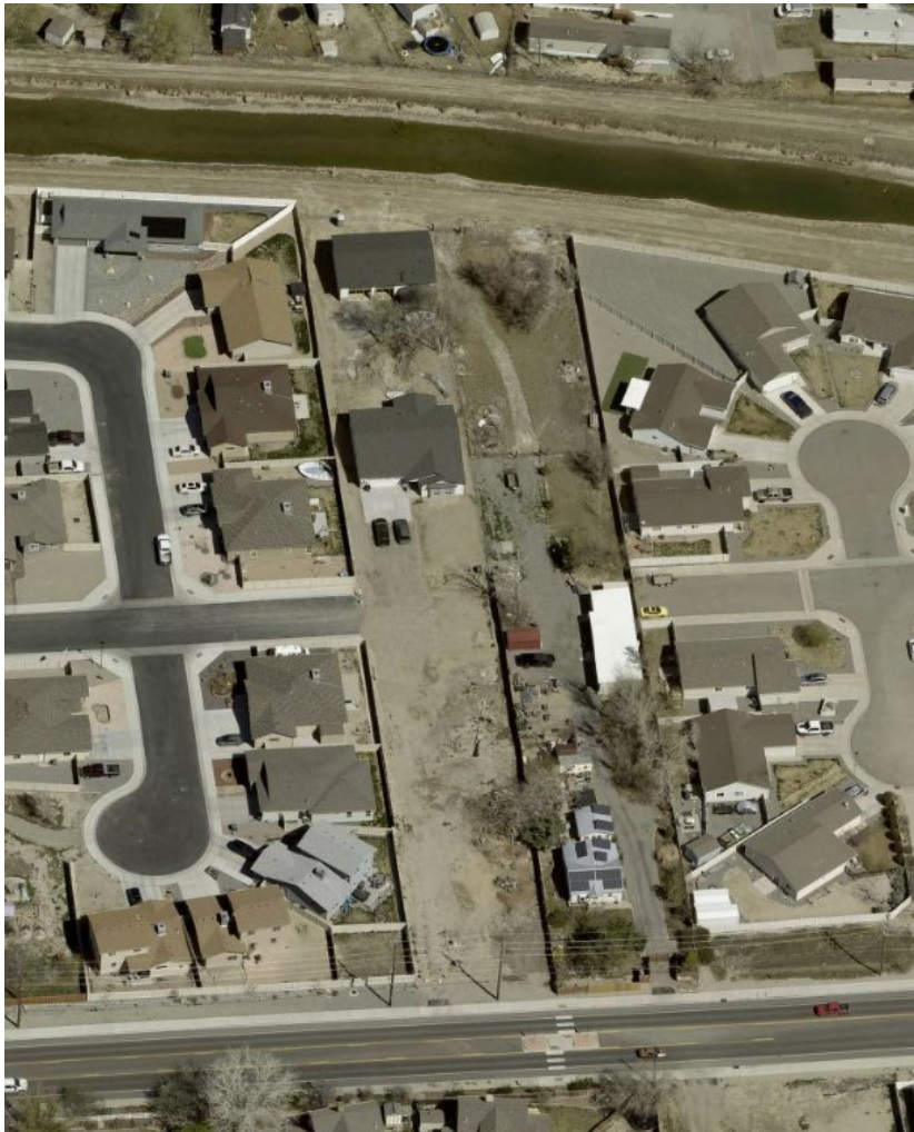
Pino Annexation – 3140 E Road – Looking north
