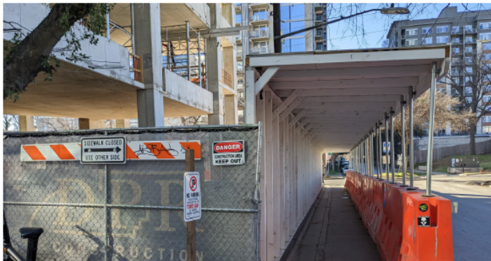
FIGURE 43: EXAMPLE OF COVERED WALKWAY AT CONSTRUCTION SITE
