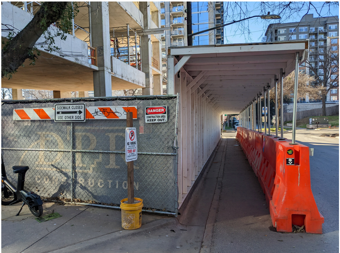
FIGURE 43: EXAMPLE OF COVERED WALKWAY AT CONSTRUCTION SITE
