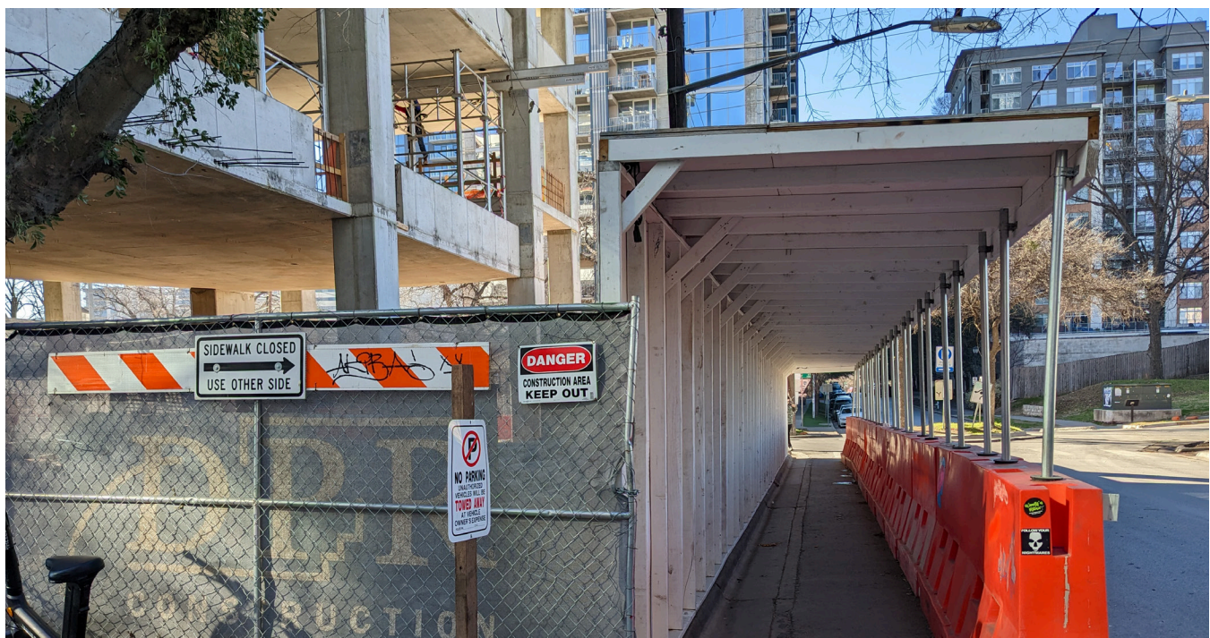
FIGURE 43: EXAMPLE OF COVERED WALKWAY AT CONSTRUCTION SITE
