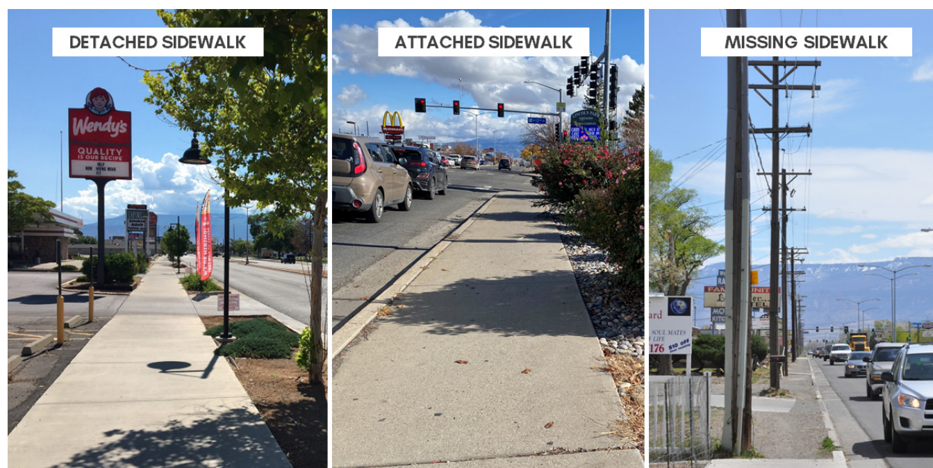
FIGURE 1: EXISTING SIDEWALK TYPES MAPPED IN GRAND JUNCTION
