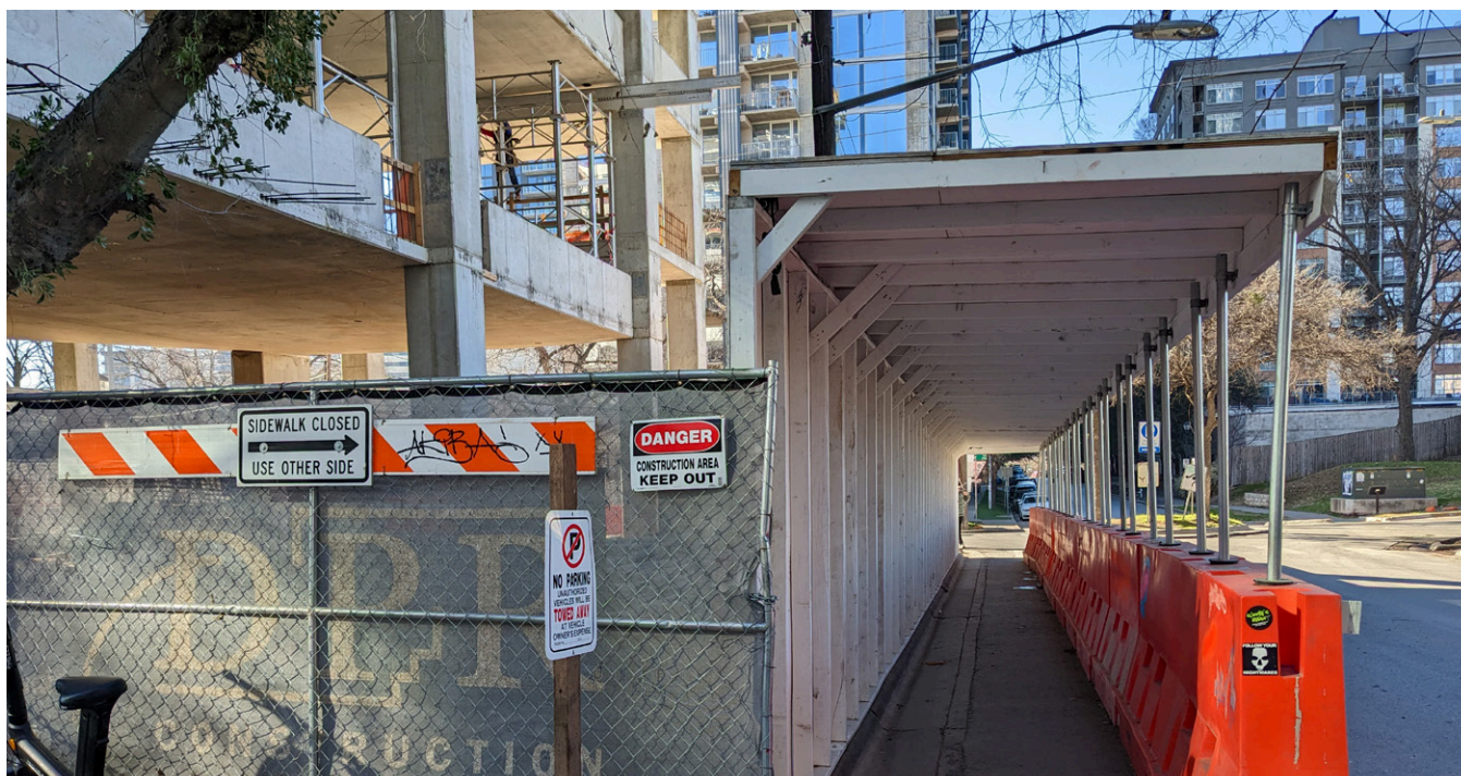
FIGURE 43: EXAMPLE OF COVERED WALKWAY AT CONSTRUCTION SITE
