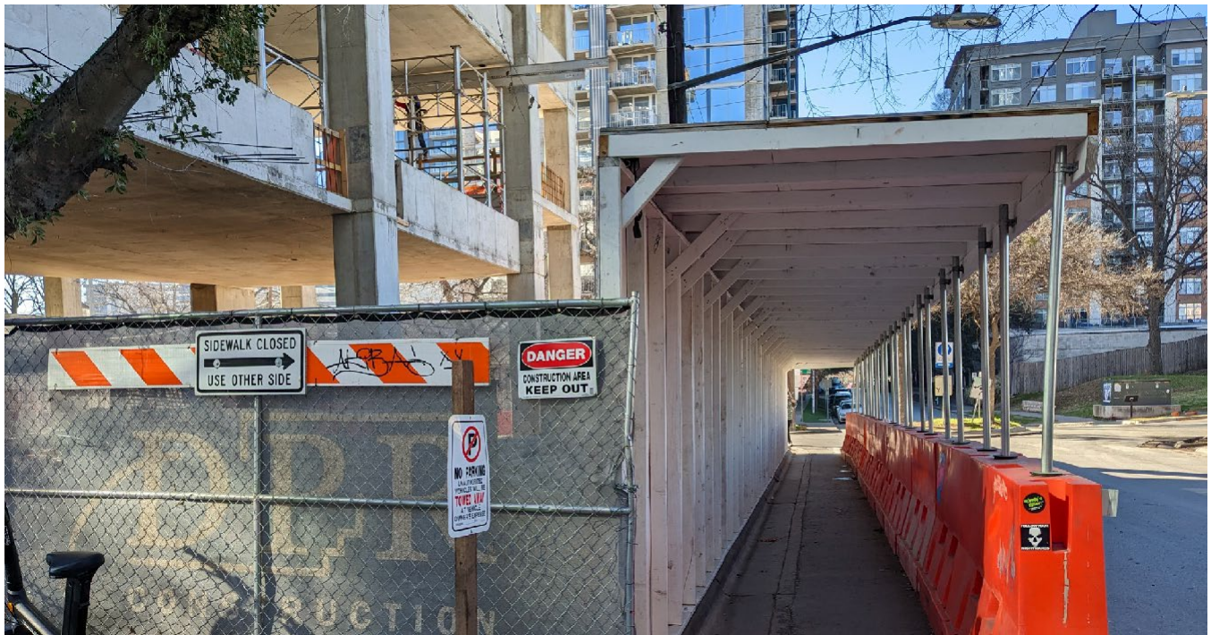
FIGURE 43: EXAMPLE OF COVERED WALKWAY AT CONSTRUCTION SITE
