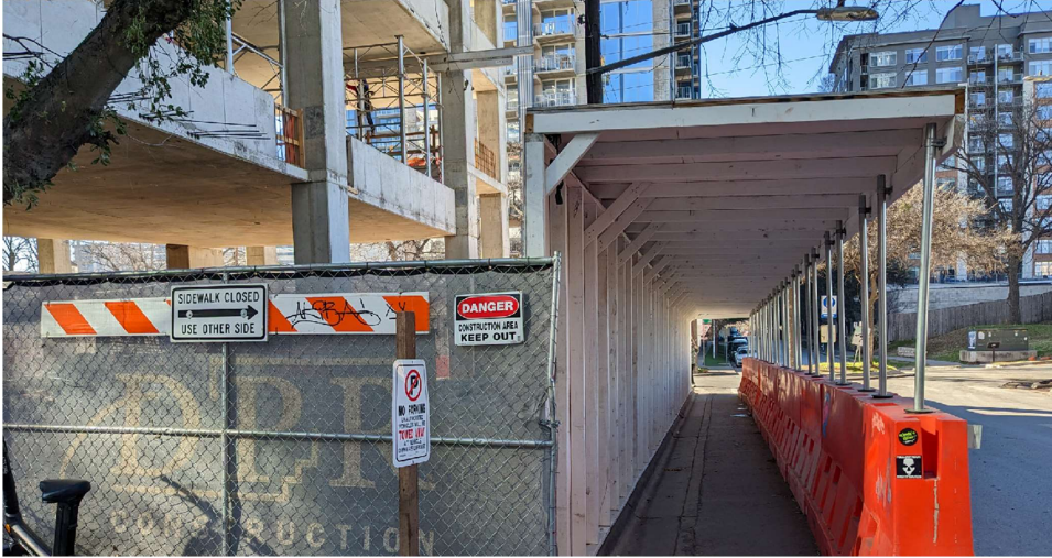
FIGURE 43: EXAMPLE OF COVERED WALKWAY AT CONSTRUCTION SITE
