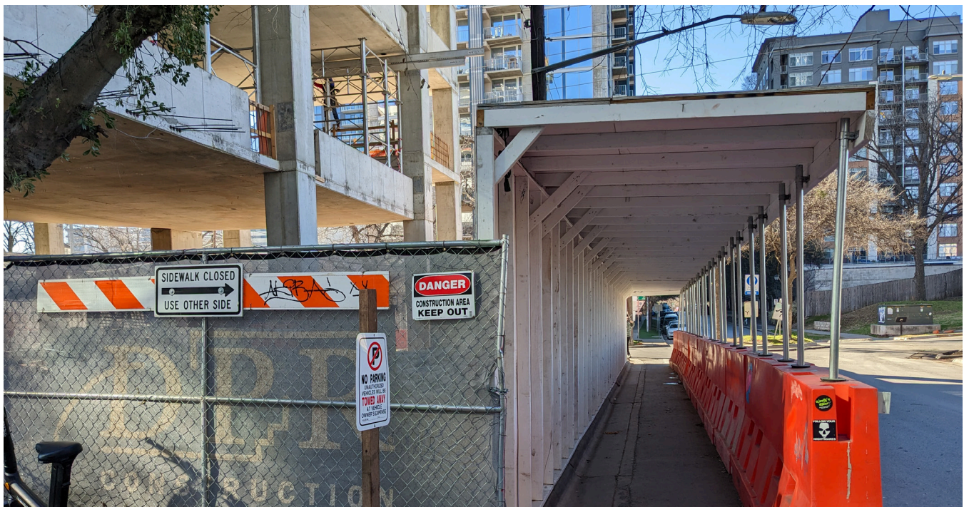
FIGURE 43: EXAMPLE OF COVERED WALKWAY AT CONSTRUCTION SITE
