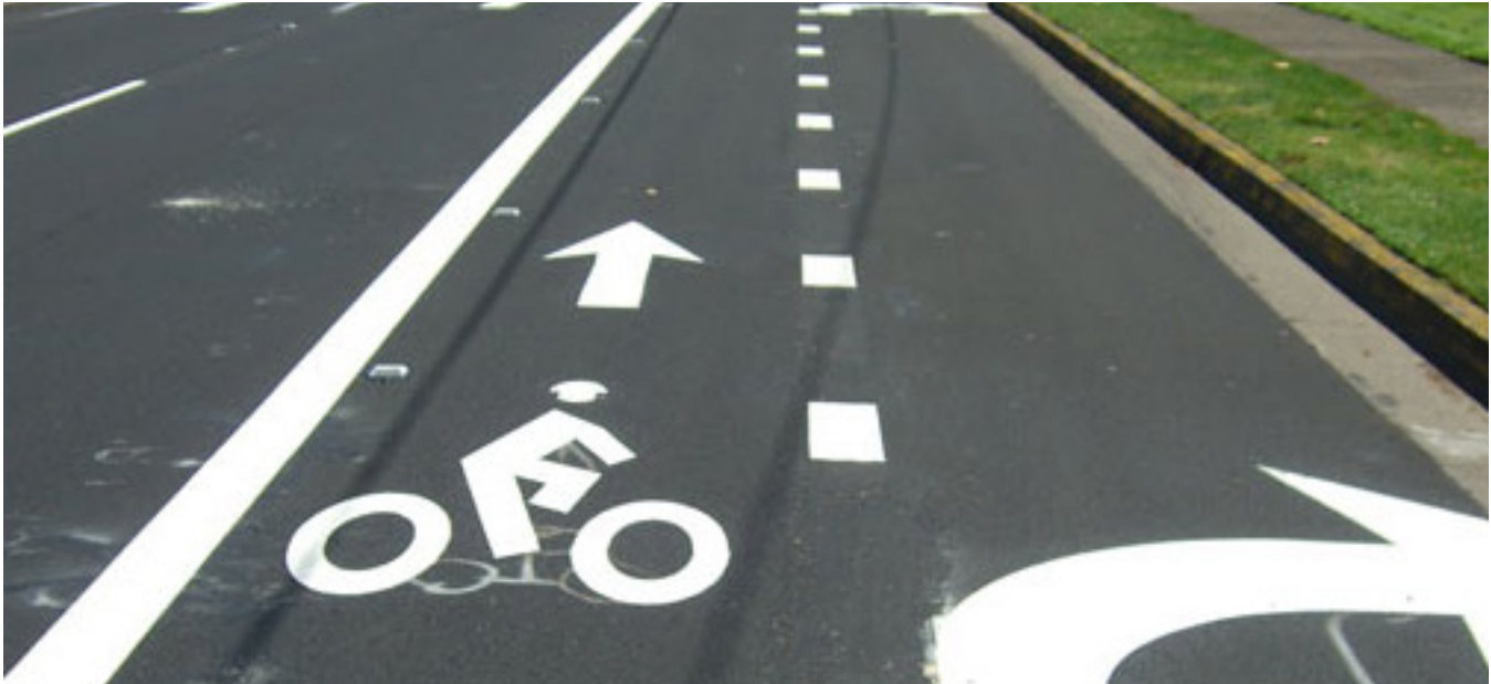
FIGURE 26: COMBINED BIKE LANE/TURN LANE
