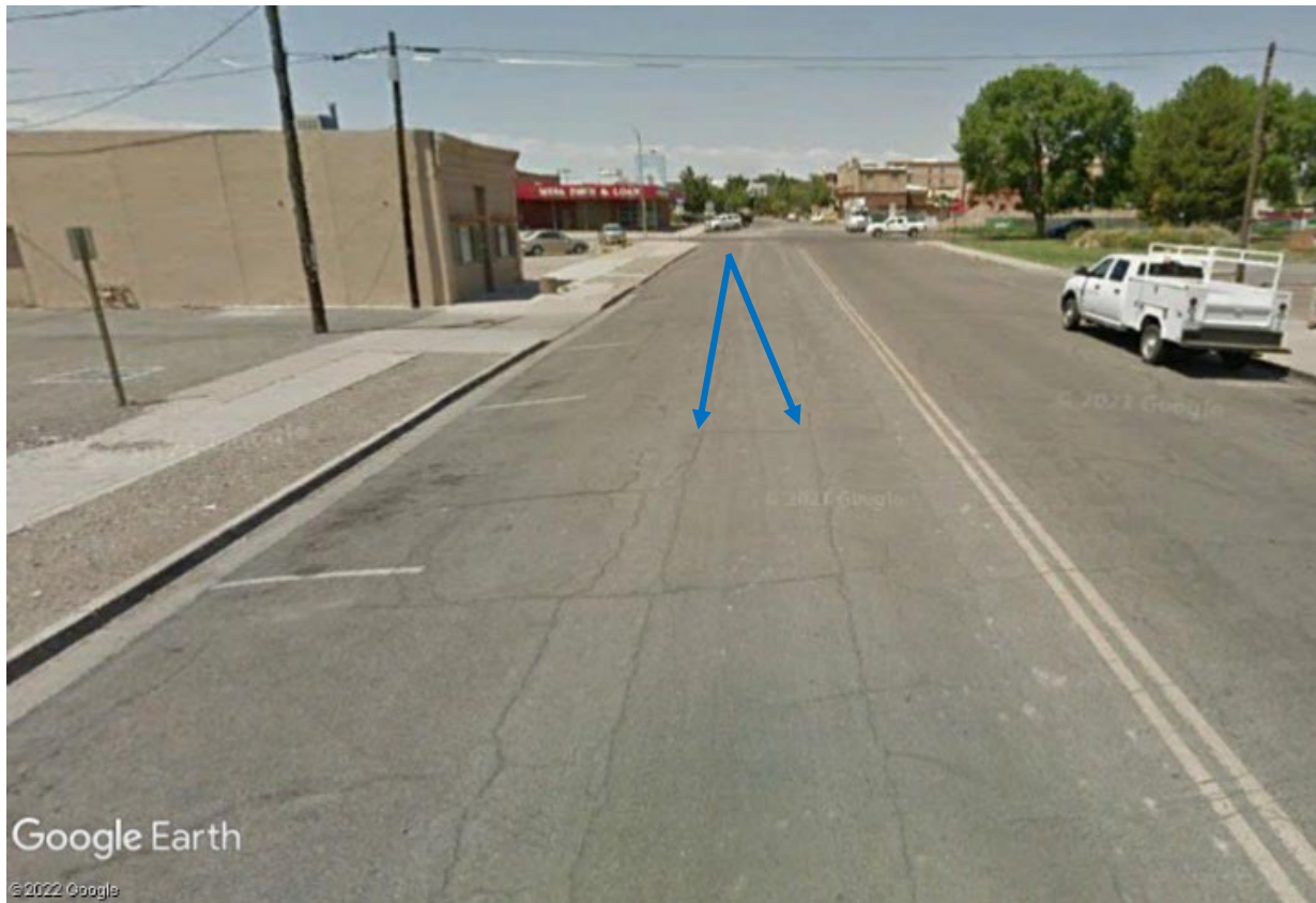
Figure 47. 5ME.24074.1. Parallel cracks can be seen in the pavement along the 300 block of 2nd Street between Ute and Pitkin Avenues. View north. Image courtesy of Google Earth.
