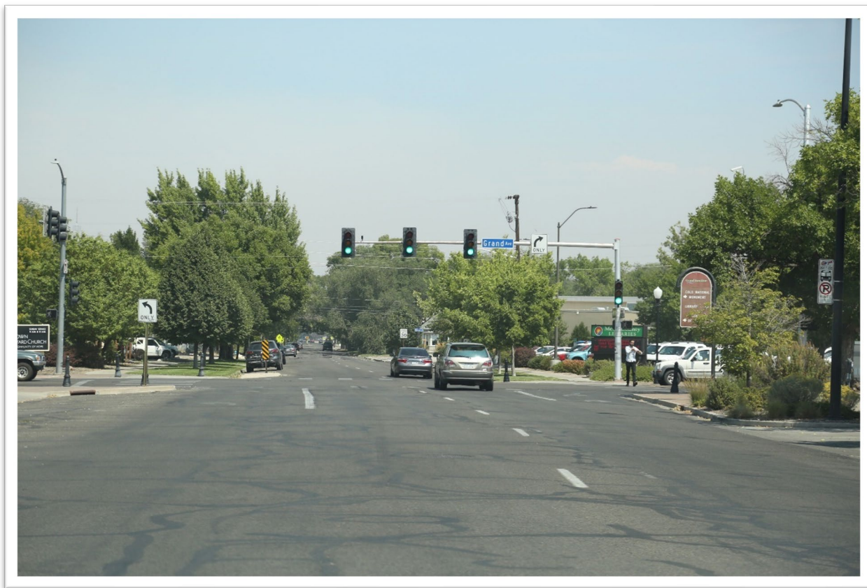
Figure 23: 5th St and Grand Ave – Looking North
