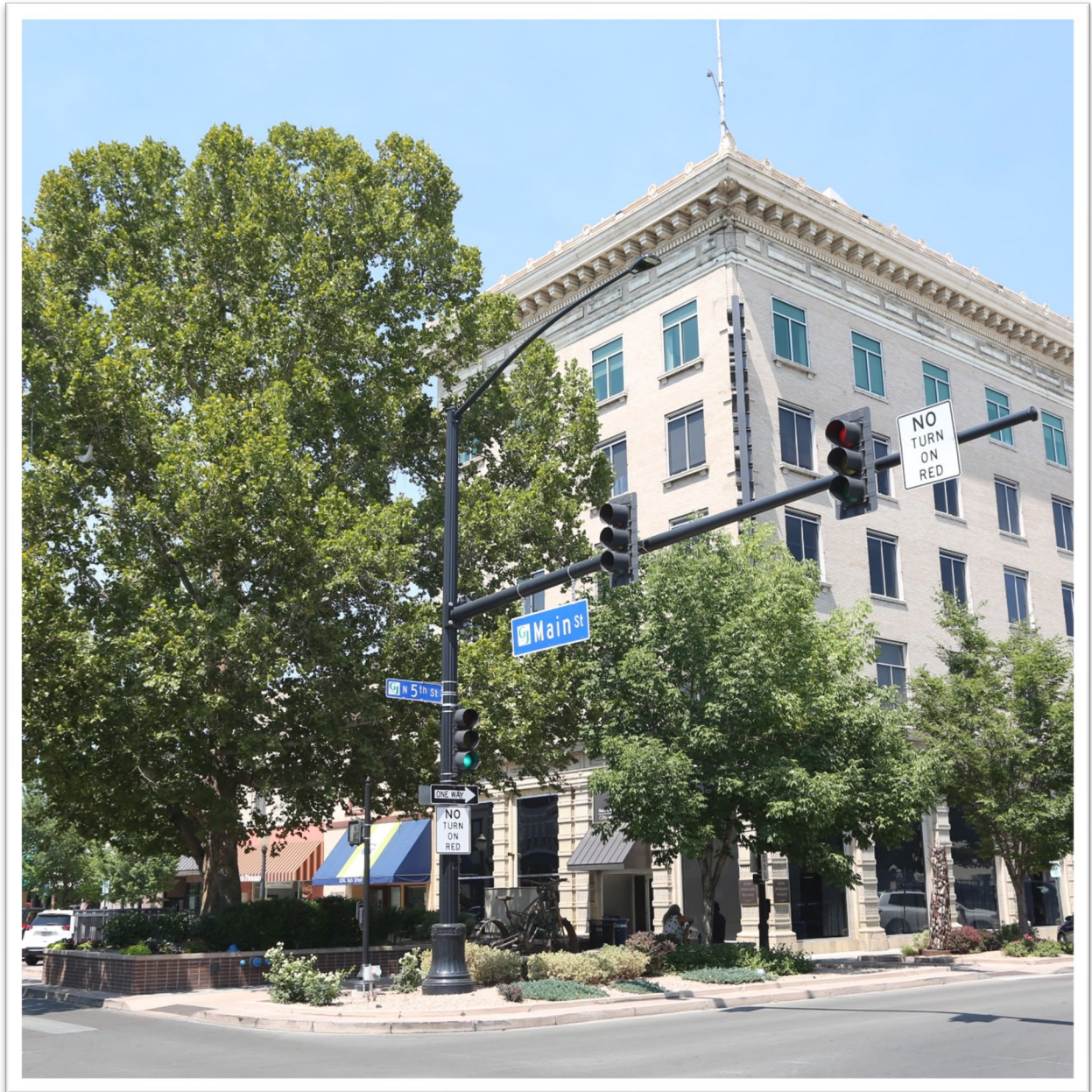
Figure 45: 5th Street and Main St – Looking Northwest
