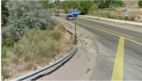
Looking NE from S. Broadway
