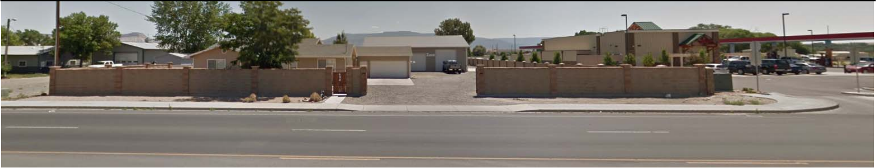
View of property from 29 Road looking east
