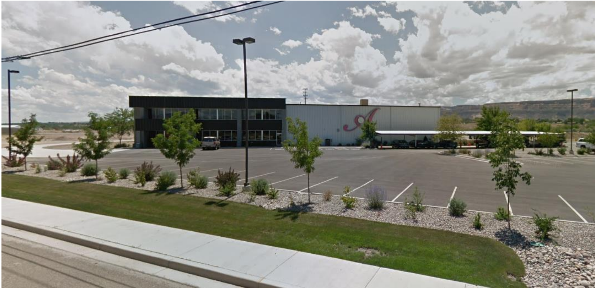
2285 River Road – Existing Building Looking South from River Road
