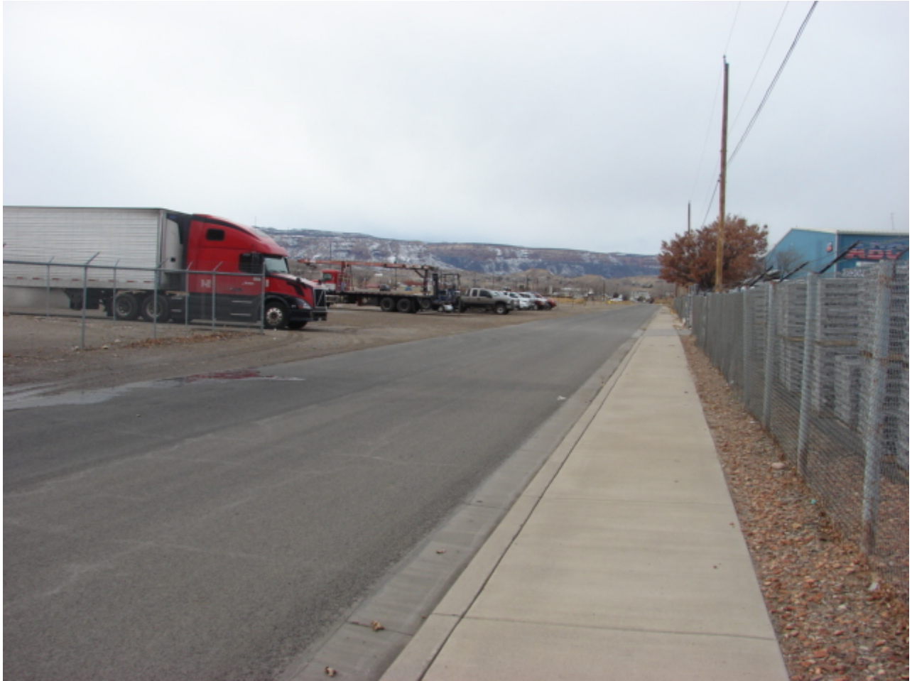
Photo 3 – Sidewalk along north side of Kimball Avenue
